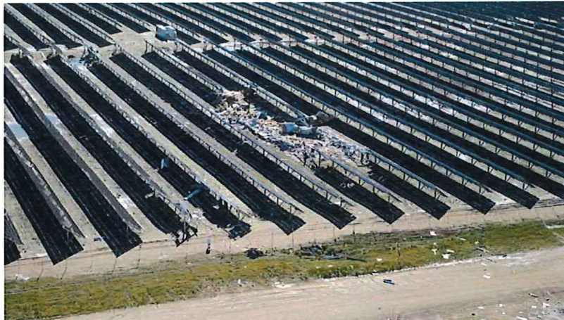
Camp Ripley received damage to multiple buildings including parts of the 60 acre solar field, built in cooperation with Minnesota Power, during a storm Sept. 7, 2016. (Photo: Staff Sgt. Anthony Housey, Public Domain)
