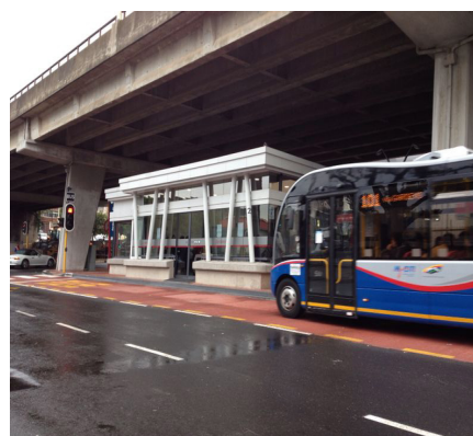
MyCiTi bus and feeder station, Gardens
