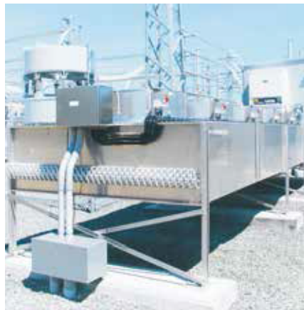
Dry air blast cooler
