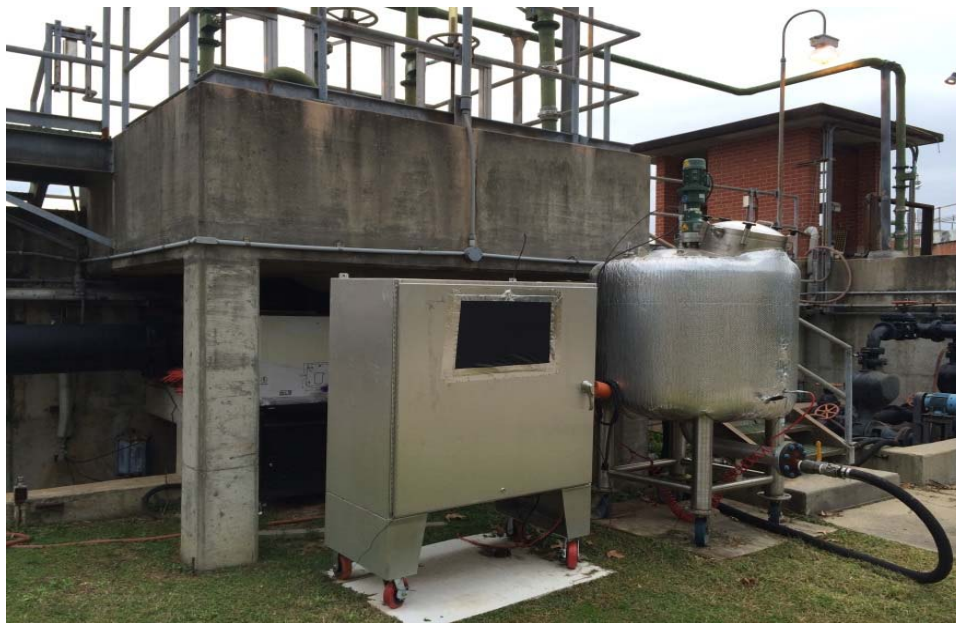
Figure 24: The pilot digester at its present location at the East Wastewater Treatment Facility in Lafayette, LA.
