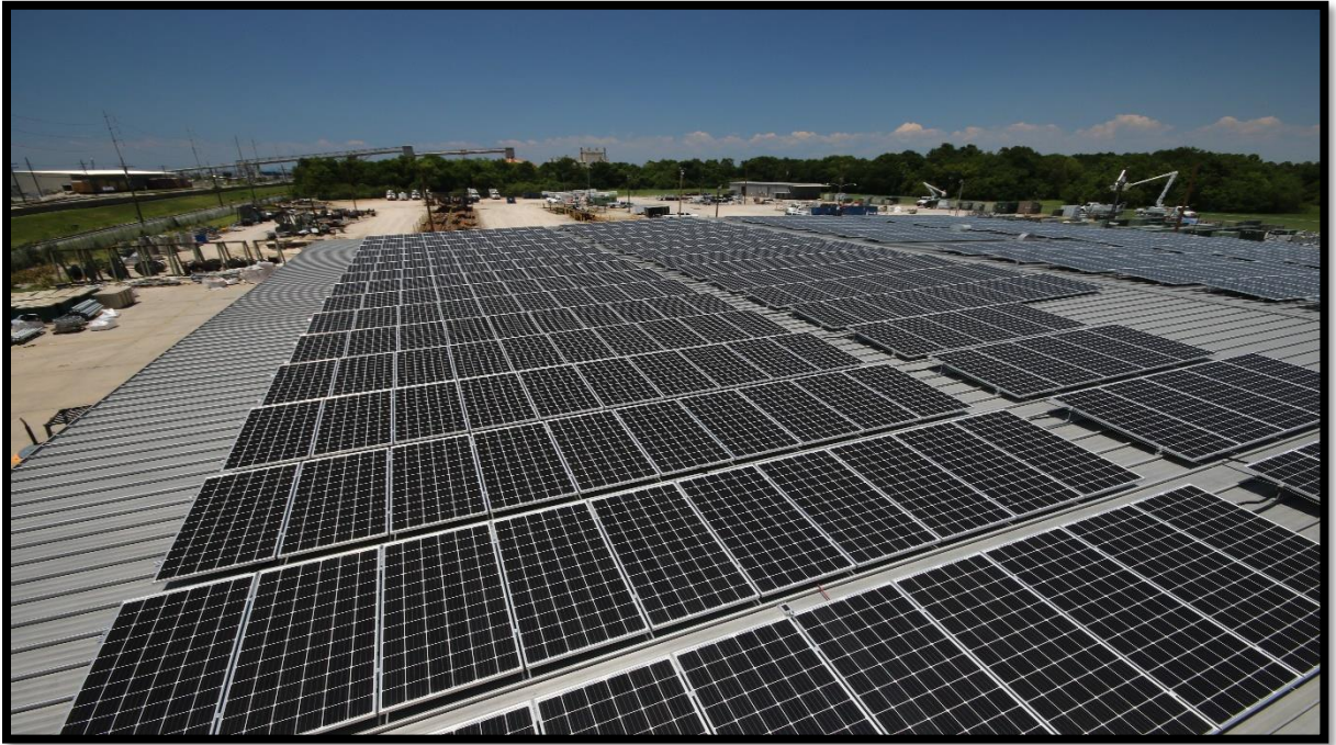
Figure 1: ENO Customer Service Center (Dwyer Road)
