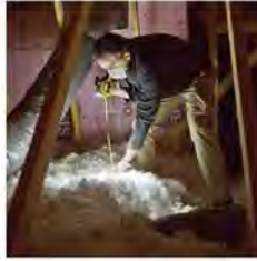
Better ventilation and humidity control
